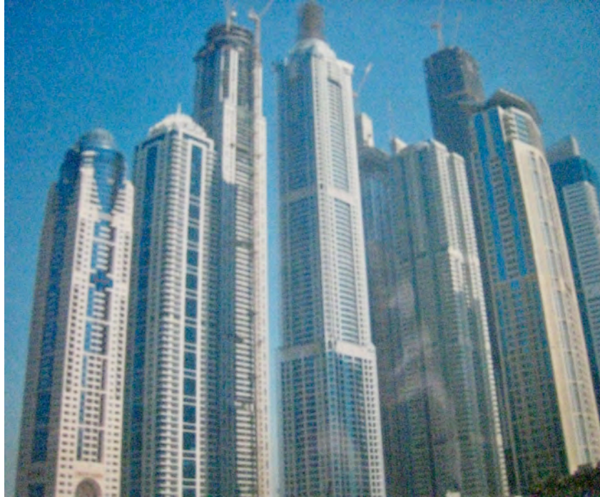
Figure 4. High-rise building in Dubai (photo by the Author)
