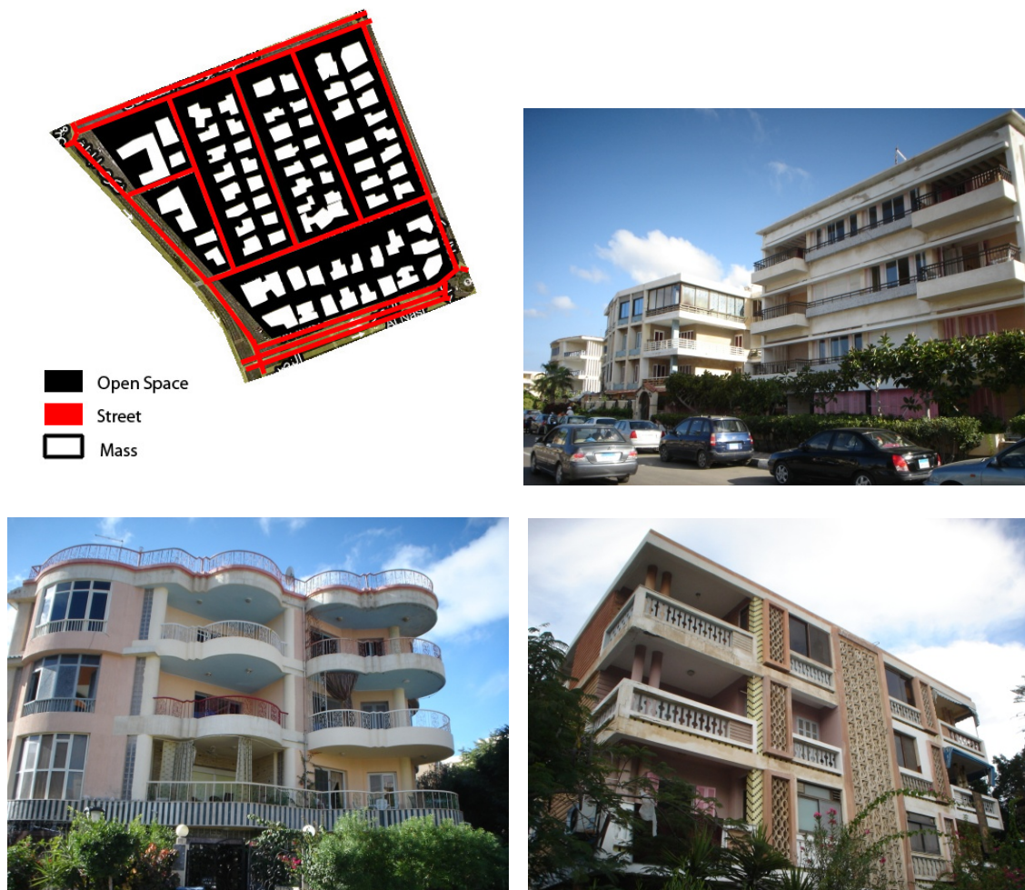
Figures 13, 14, 15, 16. Residential Block; view showing the form of buildings overlooking Youssef El Sebayi street; shape of apartments (Source: Researchers, 2010-2011)
