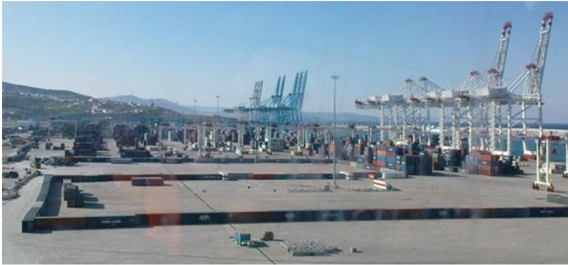
Figures 7, 8, 9. Some views of Tangier Med new terminals (credit: authors)
