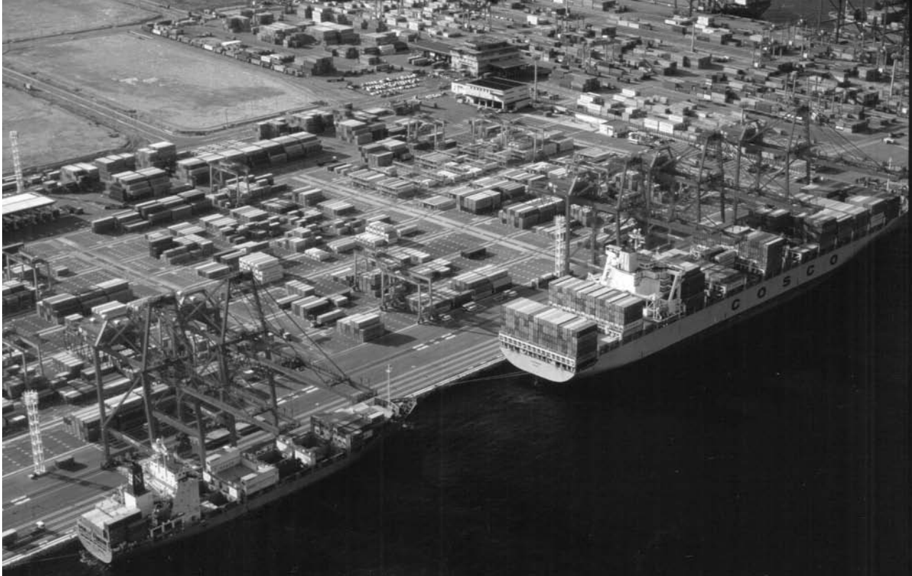
Nuevas terminales de porta-contenedores inauguradas en Port Island (2ª fase) tras el terremoto New Container Terminals Opened after the earthquake in Port Island 2nd stage
